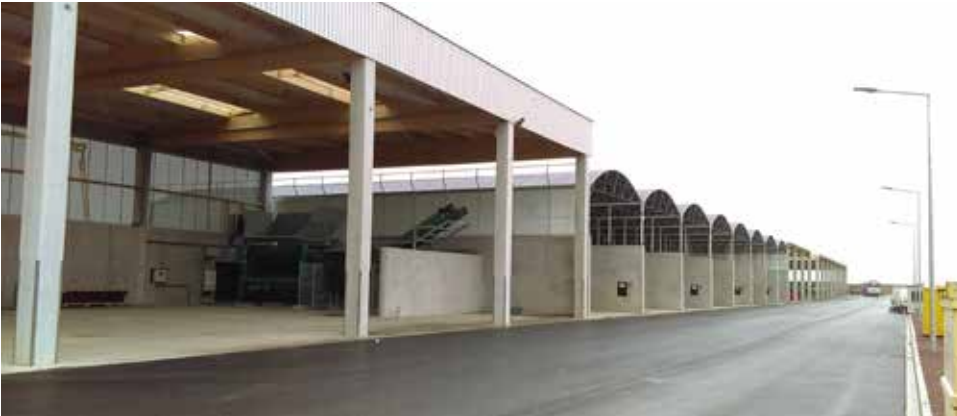
Stage 2 – Intensive composting: The shredded material is dried for three weeks in eight BIODOMES® tunnels equipped with aeration slabs and ventilation system.
