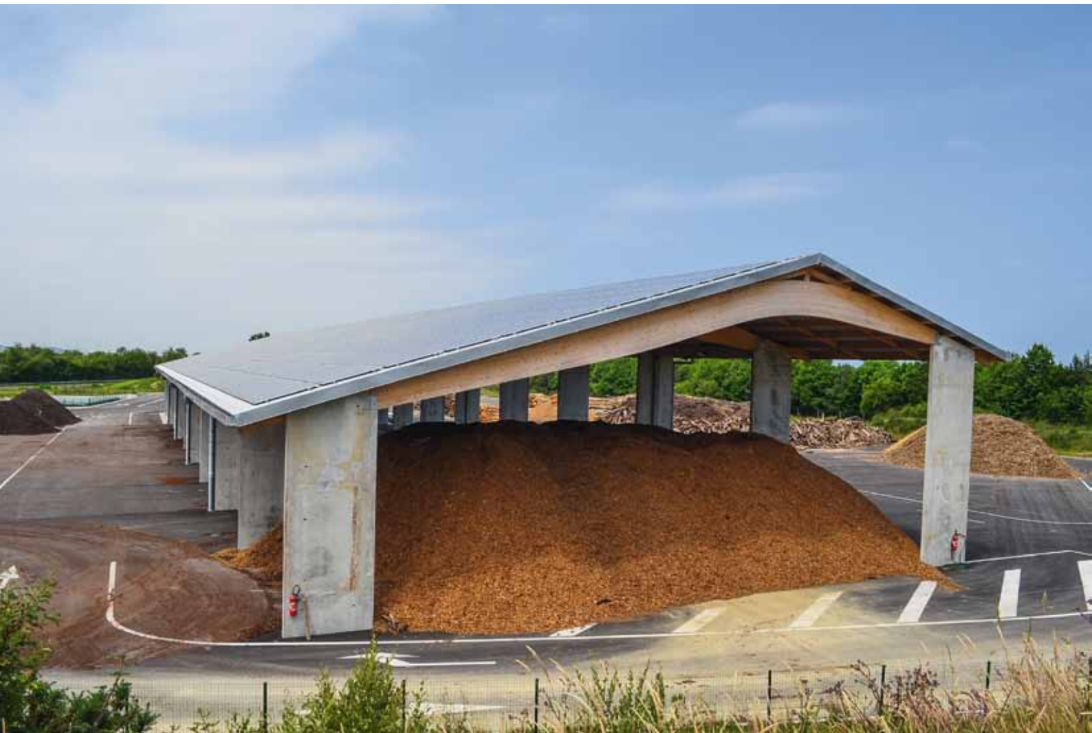
Chips are stored in a large hall.
